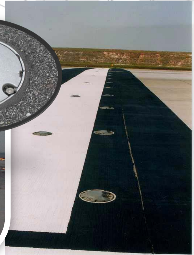
Threshold Light & End Lights
