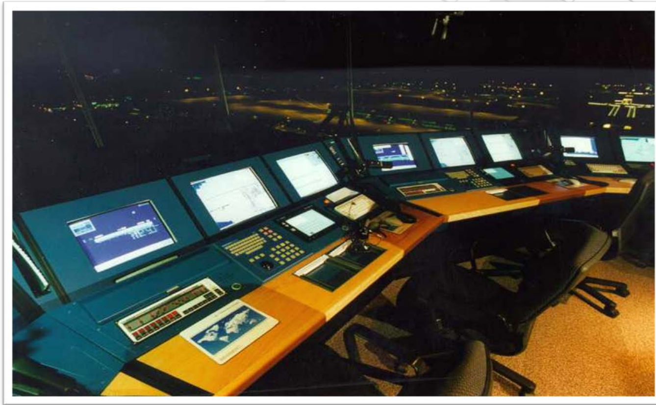
Control Tower - Controller Working Position
